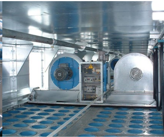
▼ Cleaning process: Purge air
